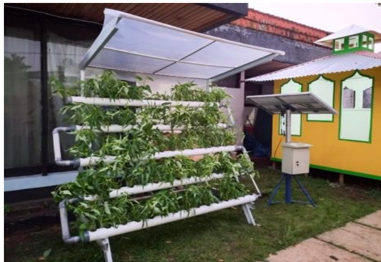
Figure 8. Installed PV-Hydroponic Integration System
