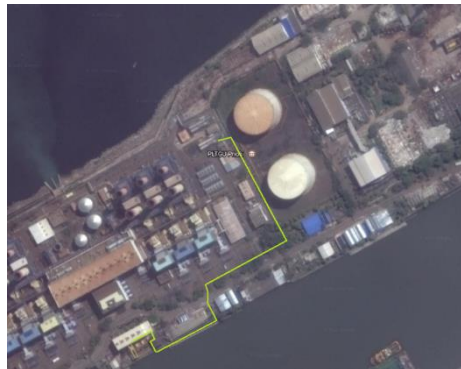
Figure 2. Head Loss Line Pipe Calculating Source: CCPP Tanjung Priok
