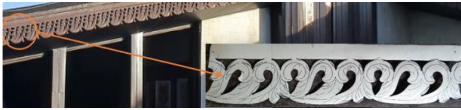
Picture 5. Slanted daun jeruju (facade): tilted units; translation vector still parallel to molding
