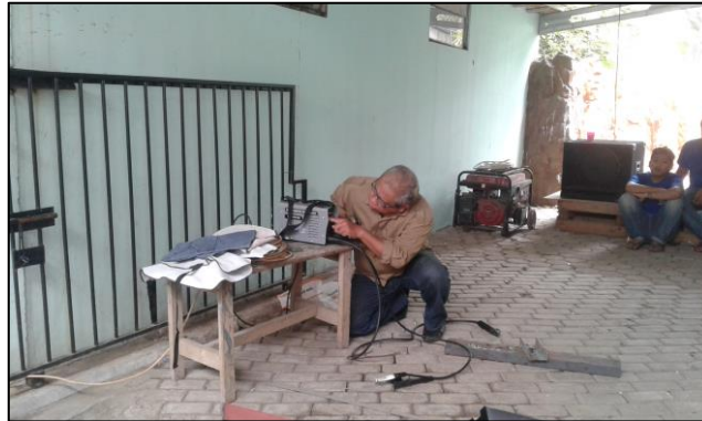
Figure 6. Installation of positive and negative welding cables
