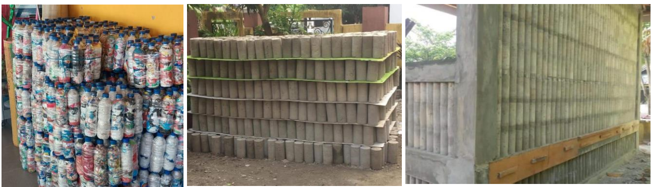
Figure 8. (a) Processing of plastic waste into ecobricks; (b) Ecobricks; (c) Literacy garden from ecobricks at SMPN 23 Pekanbaru.
