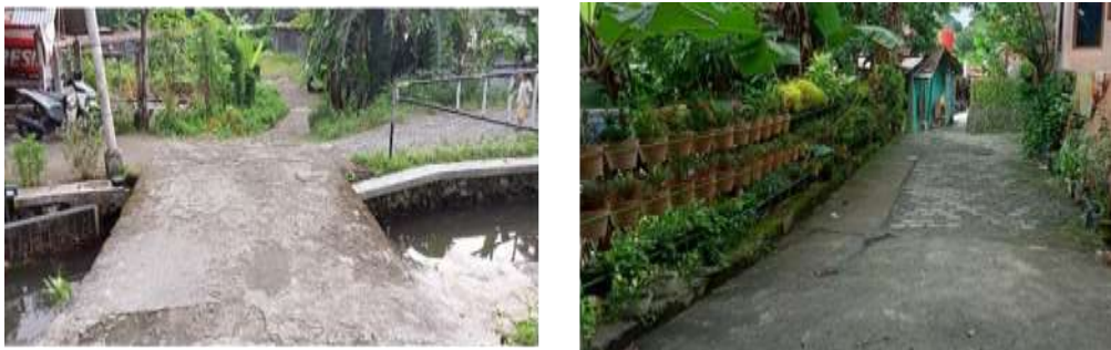
Figure 1. Physical condition of Kauman Babadan, Plumbon Hamlet
