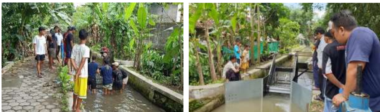
Figure 7. Submission of goods grants and installation of a mechanical bar screen device
