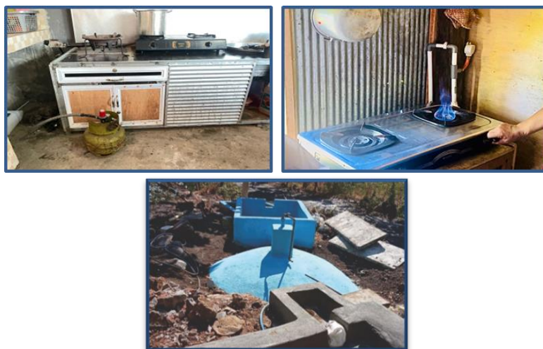
Figure 3. The installation of biogas on the stoves
