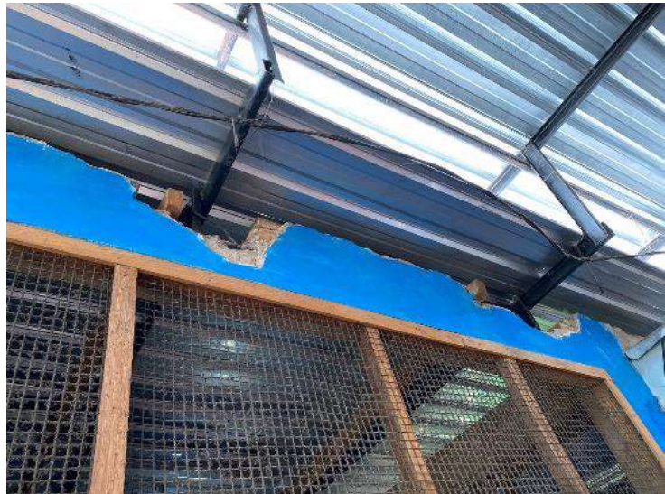
Figure 4. Market stall's wall with large opening
