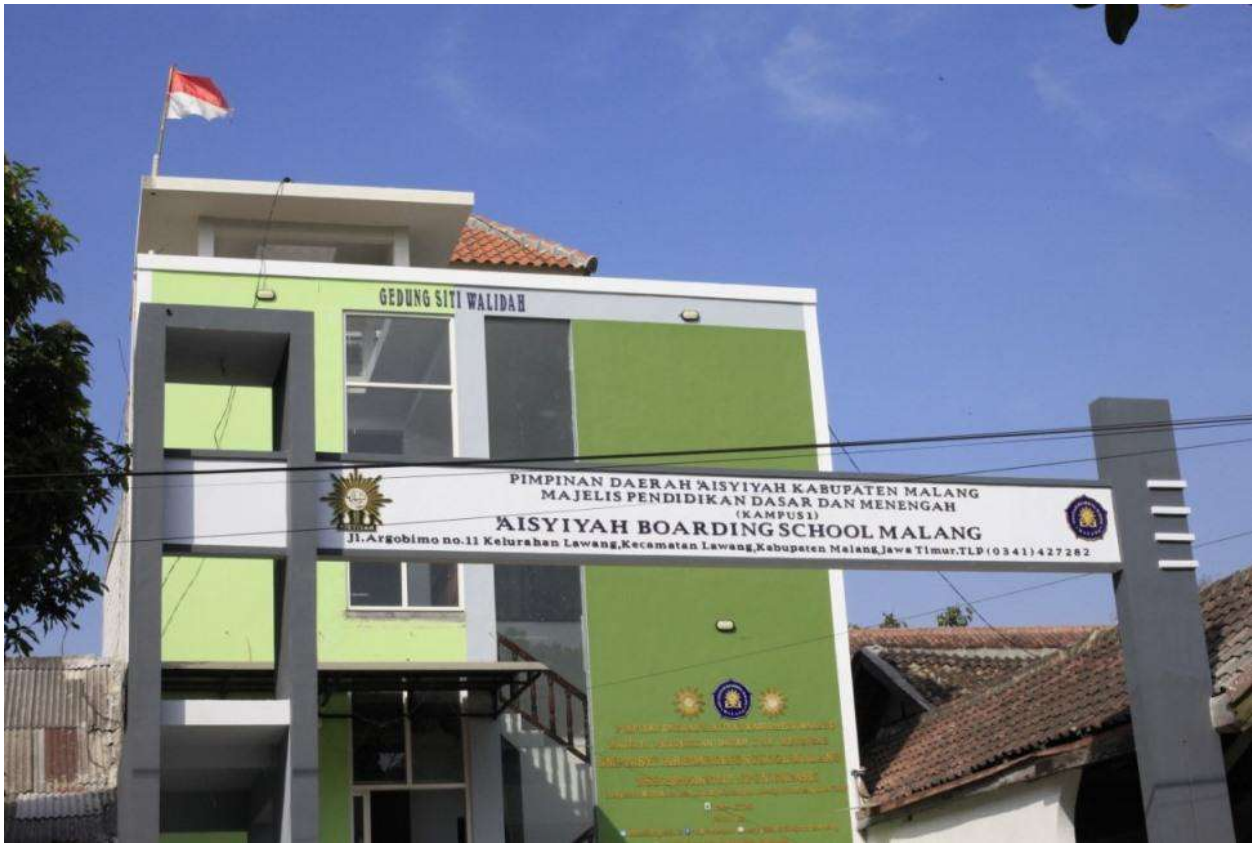
Figure 1. ABSM High School building
