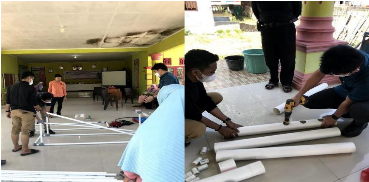
Figure 4. Training on Integrated Aquaponics and Aeroponics Installation Skills
