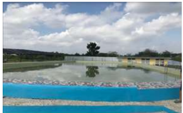
Figure 3 Waterboom Existing Condition
