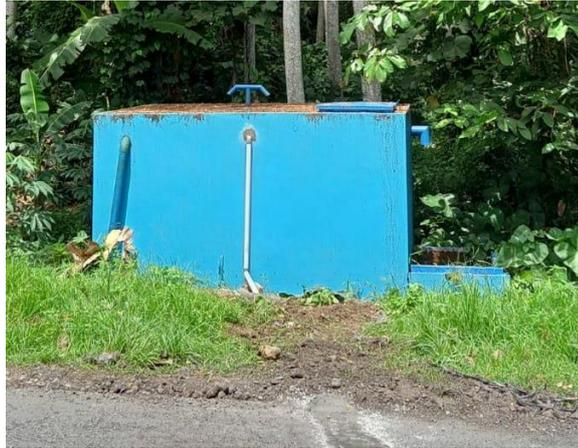
Gambar 10. Penambahan Pipa Saluran Air Dari Sumber Ke Reservoir Utama
